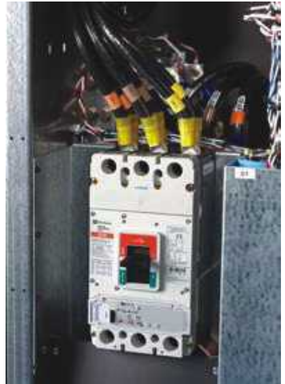
The Powerware 9395 features Cutler-Hammer LG-series input circuit breakers rated at 5 and 100 kAIC
